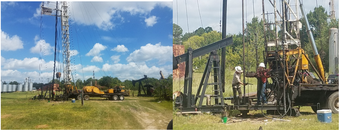
Workover rig and crew repairing the Busch H. #2B well at the Goose Creek Field
