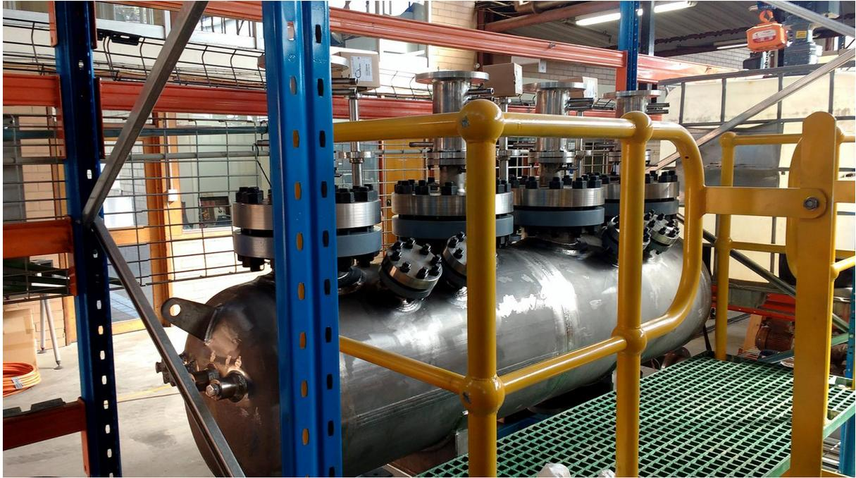
**Figure 1:** The autoclave has been installed as part of the demonstration-size plant, with commissioning scheduled to be completed in January. One of the world's leading inspection, verification, testing and certification companies completed a series of stringent quality assurance and control testing of the autoclave and subsequently certified that it complies with Australian standards.
